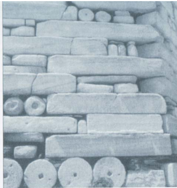
This medieval wall on the Greek isle of Poros was built many centuries ago from old mill stones and remains from ancient Greek temples.
