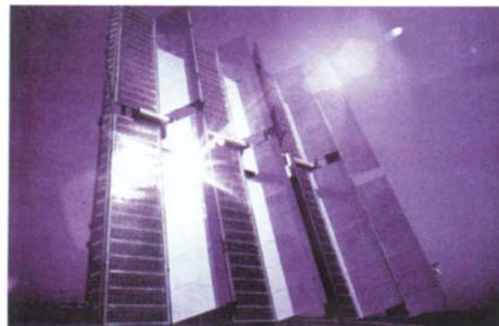
The orientation and angles of collector tilt are greatly depending on the monthly and daily solar radiation used for determining and calculating the conditions for solar collector location. The architect will have many more variants for positioning of collectors if he takes into consideration that identical values of radiation fallen on two collectors with different orientation yield solar energy at different times. The difference is smaller when the orientation is closer to pure south.
