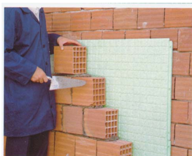
Execution of an external wall type sandwich
