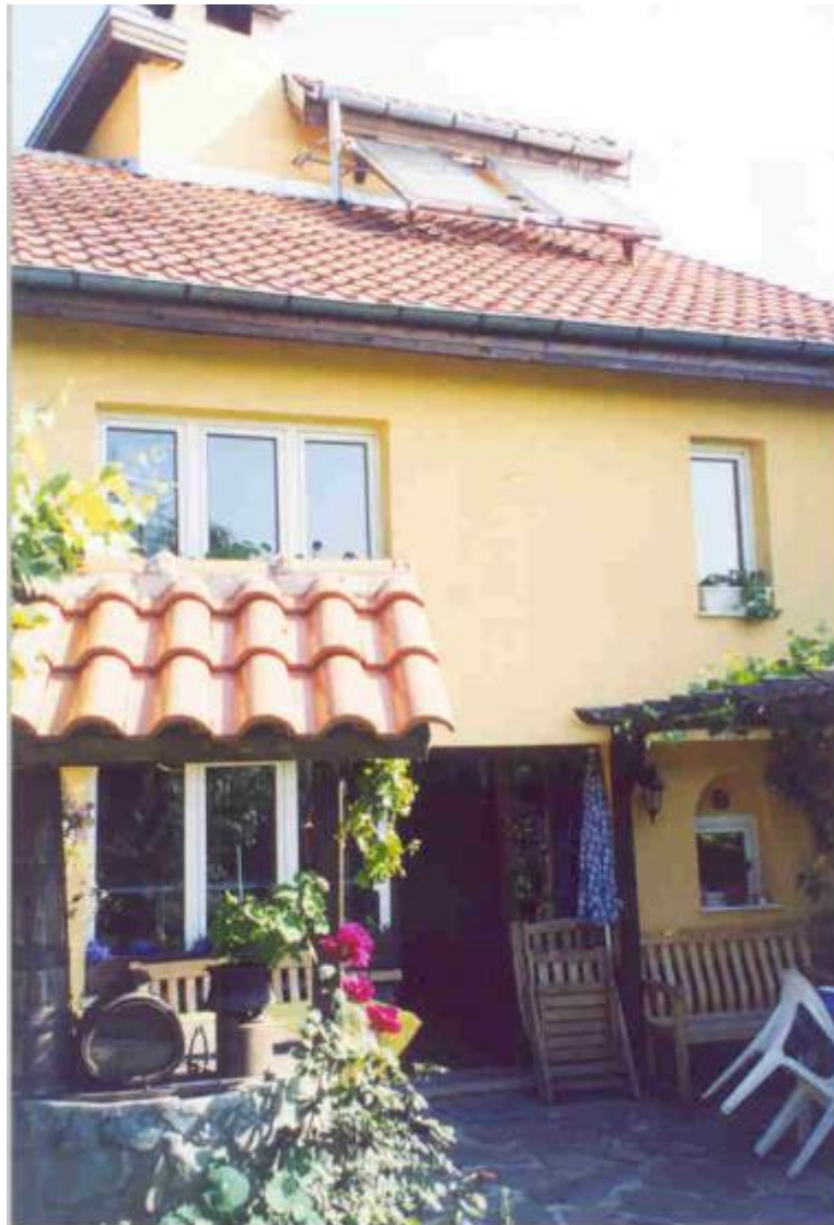
Photo 3.2 A private house in Bistrizta (near Sofia) with a pumped solar system (3,6m 2 /120l)
